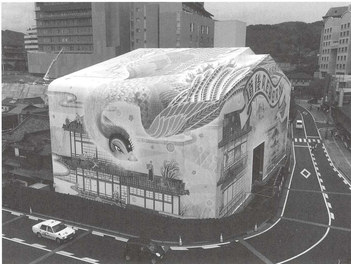
Figure 1. Dogo Onsen Honkan was closed for repairs from Jan. 2019.
